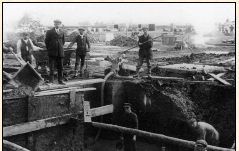
Photo right : Digging the footings © British Sugar PLC, Cantley
