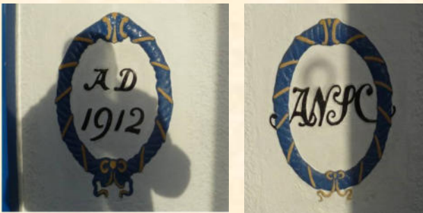
Photos: Anglo Netherlands Sugar Corporation plaques on the gateposts at Cantley.
