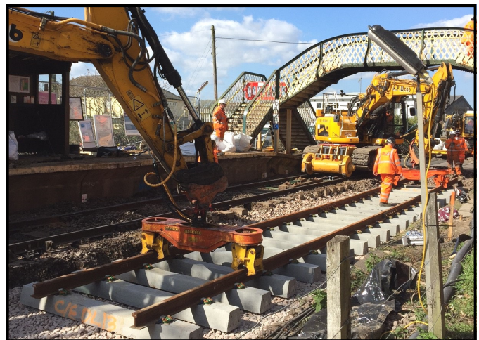
Panel Laying at Brundall Station 2019 © Network Rail
